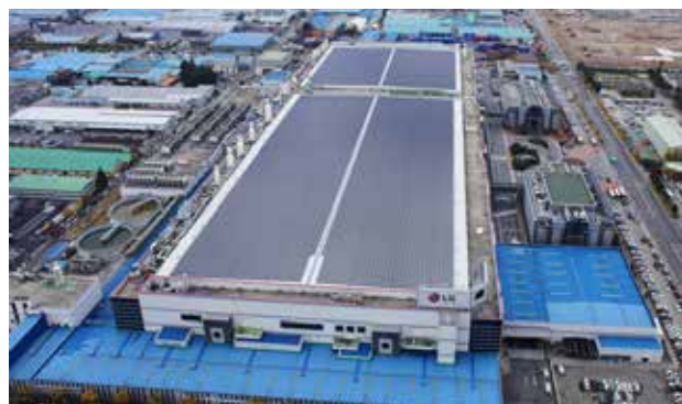
LG Solar factory, Gumi, South Korea with LG solar panels on the roof.
